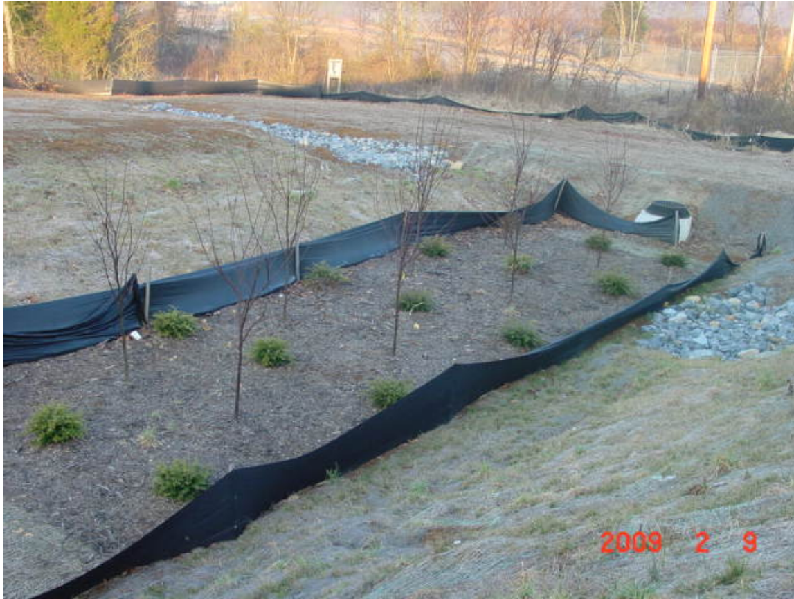
Rain garden under construction in Elizabethton.
